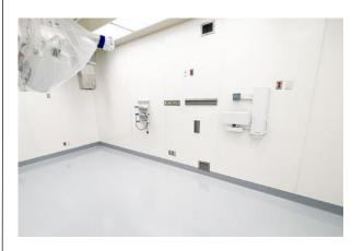
Whiterock is a material commonly used on walls in DNA clean rooms as it provides a smooth and easily cleanable surface.
